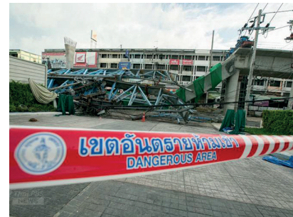
After the construction project to elevate On Nut-Lat Krabang, a collapse occurred.
