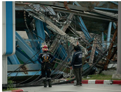
After the construction project to elevate On Nut-Lat Krabang, a collapse occurred.
